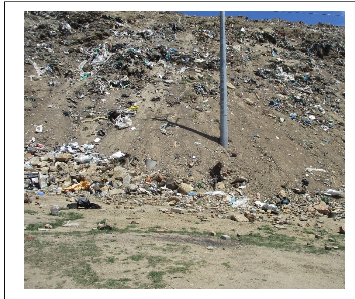
Figure 5: Waste spilling onto power line, support mast
