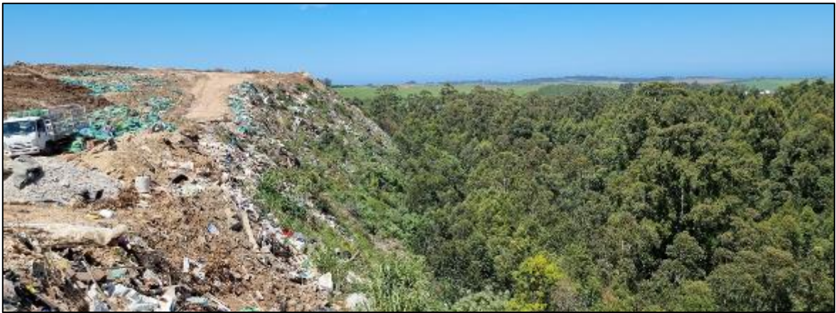
Figure 6: The steep angle created on the west face above the Gwaing River.
